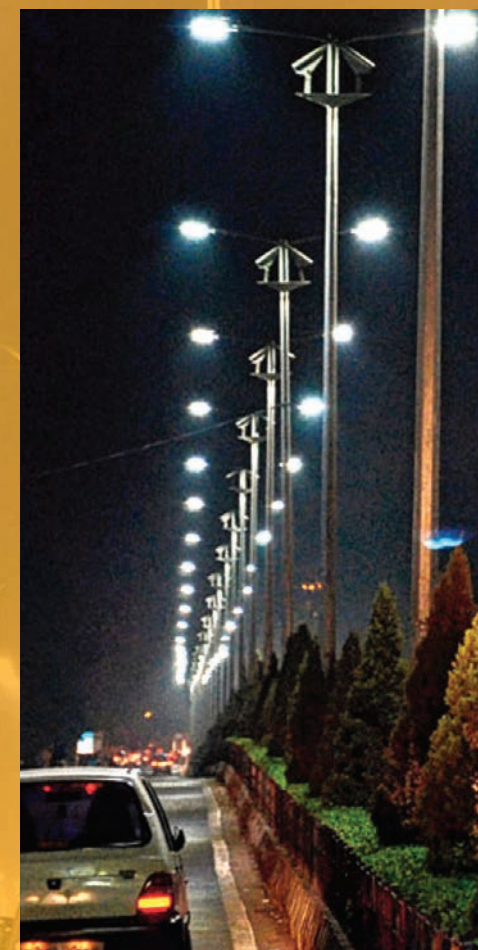
Low-carbon LED street lighting is a key part of smart city infrastructure and helps combat climate change
