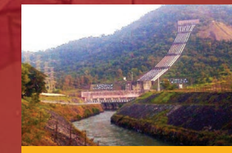
Small and medium hydroelectric plants provide clean energy
