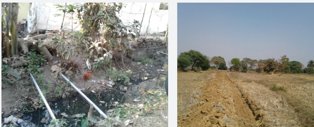
FIGURE 30: (a) View of minor 6c of distributary no-6 of Kendrapada canal in deteriorated condition; (b) View of tail reach of Champamal minor Hariharjore (Medium Project)
