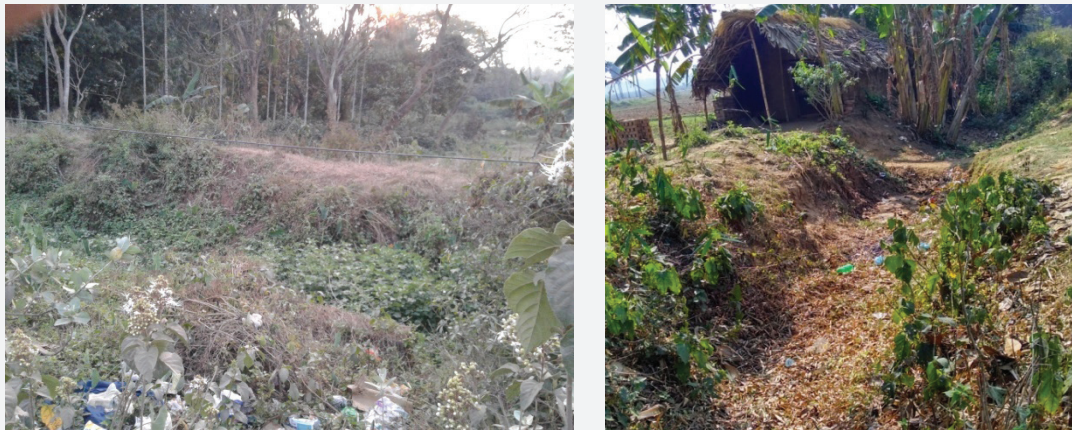
FIGURE 29: (a) View of tail reach of Rampa minor of L1 distributary; (b) View of tail reach of 8H minor of distributary no.8 (Kendrapada canal)
